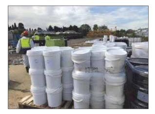
**Fig. 6**. ELS<sup>®</sup> Microemulsion component in 200 L steel drums, and EHC<sup>®</sup> Liquid mix component in 11.7 kg bags delivered in plastic pails
