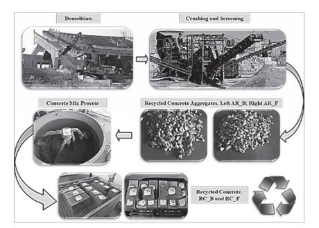
Fig. 2. Demolition of Sant'Elia Stadium concrete structures, RA and RC obtained
