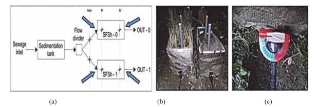
Fig. 3. Pilot plant scheme with flow rate measurements points identified with blue arrows (a). SFSh-0 and SFSh-1 tanks view from the output (b). Detail of the regulation valves(c)
